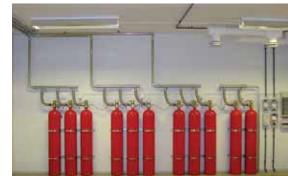
Computer room at University of Lund Sweden: Library protected with Clean Agent FS 49 C2
