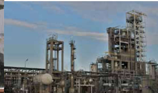
Petrochemical Industries: Laboratories, High Risk Areas and Storage Rooms protected
