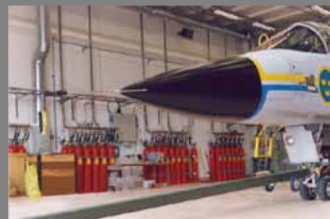
JAS 39 Gripen: The Swedish Airforce's latest multi-role fighter, hangar protected by 7000 kg FS49C2
