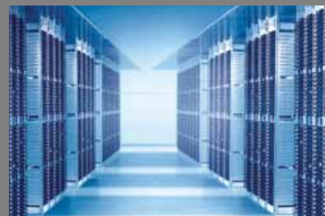
Server and control rooms: Provided with rapid fire protection that does not damage equipment, it just quickly takes out a fire.
